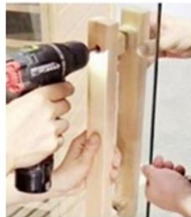
2. Install the handle, screws from the inside of the sauna.
