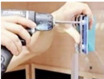
1. Install the hinges - the soft parts must be next to the glass, on the inside of the hinges 2.
